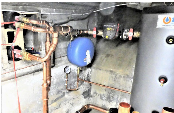
June 2022 Jupiter connect pipes in the boiler room:
